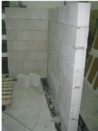
Figure 1. View of the wall before plastering.
