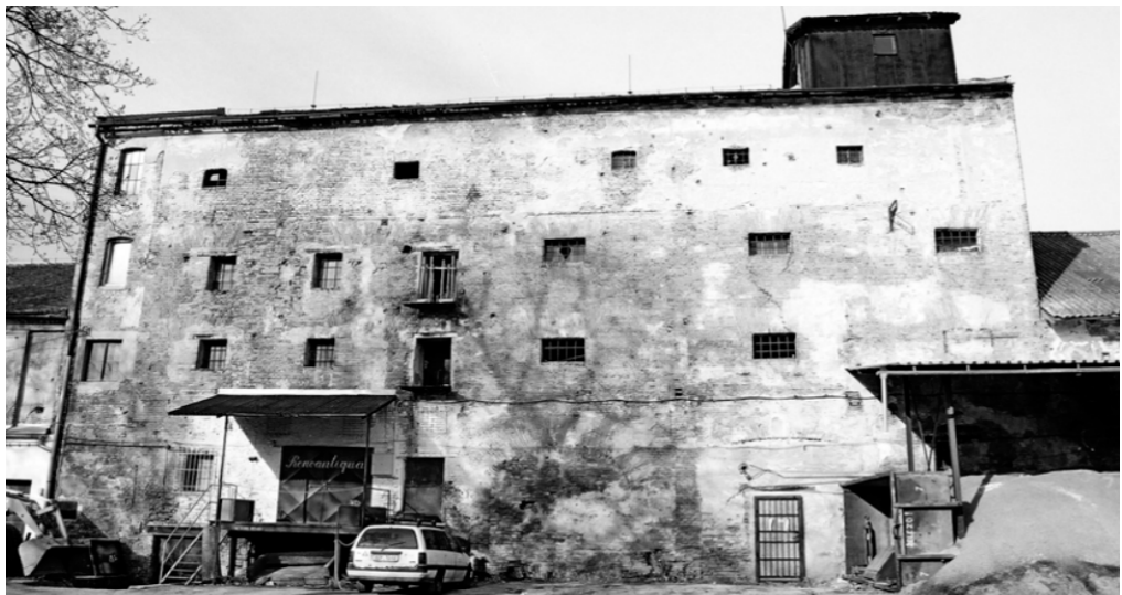
Figure 6. View of the courtyard facade of the former malt house; source: [53].
