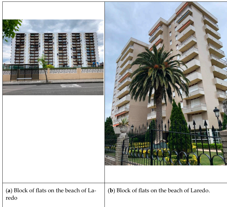
Figure 13. Residential construction around Salve Beach (Laredo). Source: own images.
