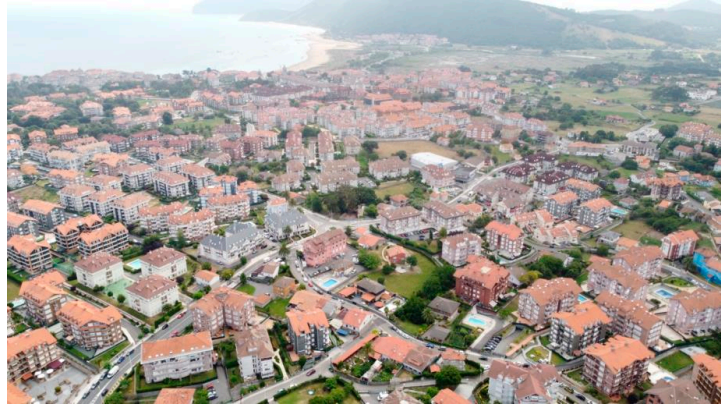
Figure 12. Residential construction in Noja. Source: own images.
