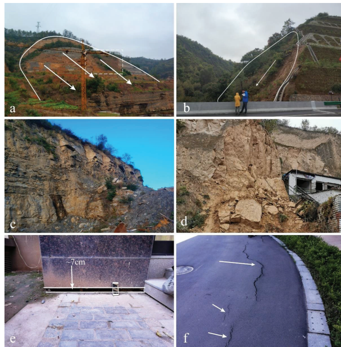
Figure 6. Examples of geohazard types mapped in the study area: (a) loess–bedrock interface landslide; (b) loess landslide; (c) soil–bedrock unstable slope; (d) soil unstable slope; and (e,f) cracks and damages in the ground and buildings due to land subsidence. Arrows indicate the direction of the slide and the location of the cracks.
