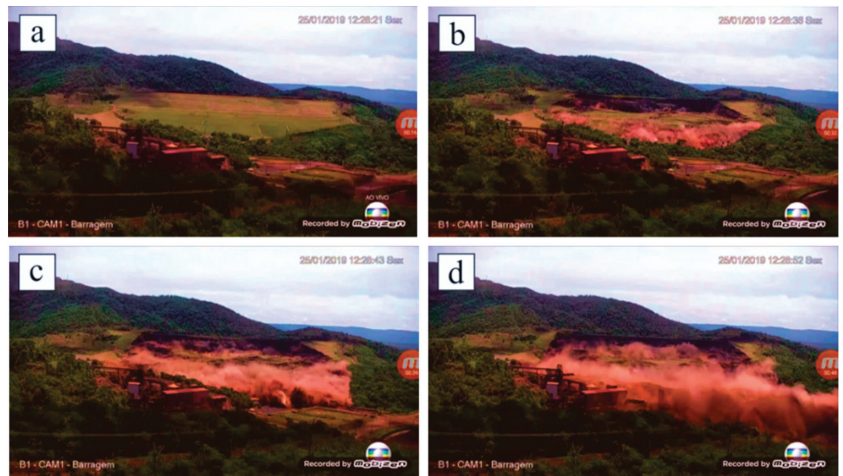
Figure 2. Video screenshots of the Brumadinho tailings dam failure [14]; (a) 25 January 2019, 12:28:21; (b) 25 January 2019, 12:28:36; (c) 25 January 2019, 12:28:43; (d) 25 January 2019, 12:28:52 (local time).
