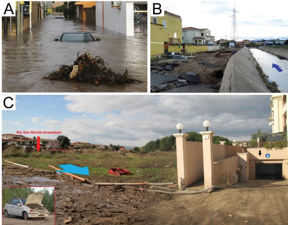
Figure 9. (A) Olbia: Although about 15 h had passed since the paroxysmal phase, in some morphologically depressed areas of the city the water remained well above 1.3–1.4 m in height. Some cars were totally submerged in one of the streets most affected by the flood in the Baratta quarter (courtesy of private citizen). (B) Olbia, left bank of the Rio Seligheddu Stream, canalized stretch (foto Luino). Water level left a marker on the wall, which is evidenced by white line. The height of the waters is evidenced by the bed dragged and placed over the roof of the ground floor (white arrow). (C) Olbia: very common situation along the areas close to the streambeds (foto Luino). In this image, the Rio San Nicola (red arrow) waters exceeded the natural bank that was devoid of embankments or retaining walls and easily reached the houses located on the left bank, which was a short distance away. In many houses, the underground garages have been foolishly built and had been totally flooded (black arrow indicates the level), with serious damage inducted to parked cars. The extracted cars are so saturated with fine material (silt and clay) that they had to be demolished (image in the left corner).
