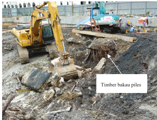
Figure 2. Timber bakau piles used as support system for the demolished buildings.
