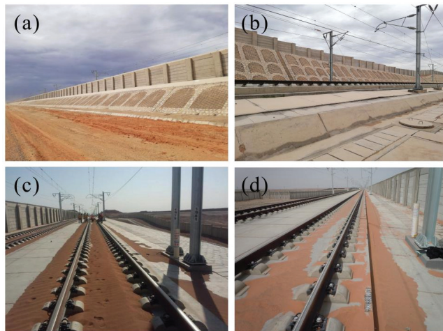
Figure 1. (a) Convex subgrade and (b–d) concave subgrades. Note: The wind-break wall is different from the sand fence (see Appendix A).
