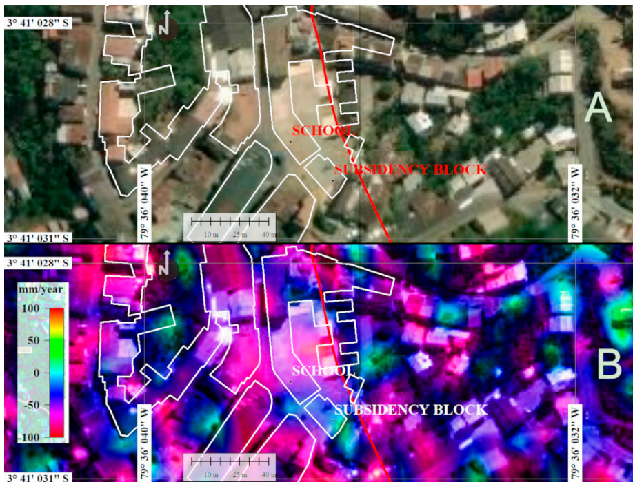
Figure 9. (A) Location of Fe y Alegría-La Inmaculada School in the study area before the collapse of the block of school classrooms. (B) Block collapse of school classrooms on October 25 of a day before the collapse that began on October 16, 2016, and completely collapsed in December 2016. The faint blue color indicates that before October 25, 2016 the sinking of the area was in process. Gallery is in red color and blocks houses are in white color.
