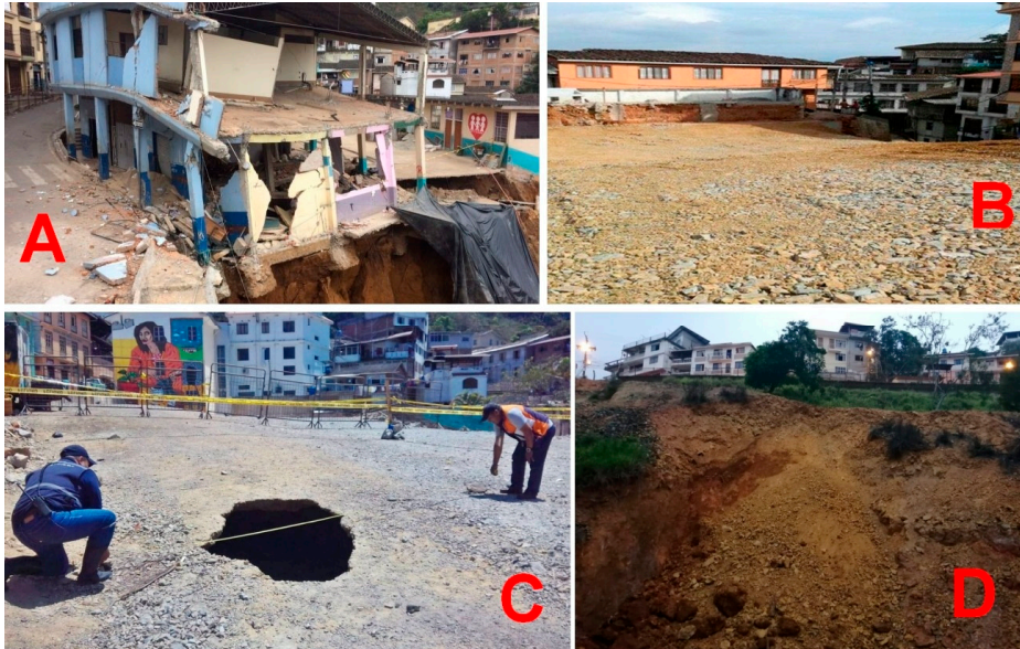
Figure 3. (A) Collapse of the Fe y Alegría School, in October 2016. (B) Technical filling done at the site in 2017. (C) Reactivation of the collapse in the place where the school was in 2017. (D) New collapse near Gonzalo Pizarro Street in 2019. Images taken from El Expreso Newspaper, Ecuador en vivo, Pichincha Universal and Arden los Socavones Facebook page.
