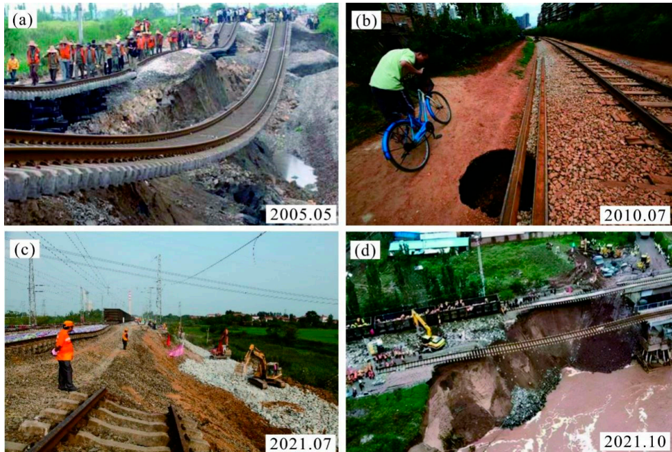
Figure 1. Typical high-speed railway foundation settlement disasters in China: (a) Xiaoyong railway collapse disaster; (b) Kunming railway collapse disaster; (c) Longhai railway collapse disaster; (d) South Tongpu railway collapse disaster.
