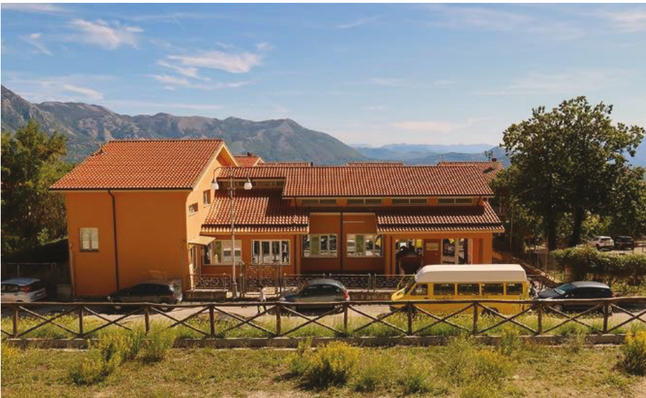
Figure 99. Senerchia: new school complex (photos by [35,36]).
