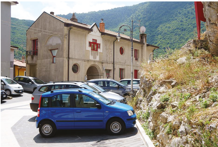
Figure 42. Balvano: the new buildings details of the architecture by R. Boffo and K. Eibl (photos by [35,36]).
