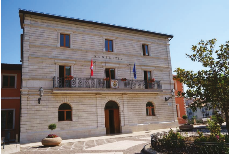
Figure 68. Pescopagano: the new Town Hall of village (photos by [35,36]).
