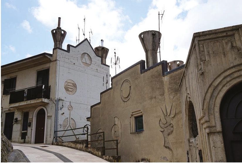
Figure 43. Balvano: the new buildings details of the architecture by R. Boffo and K. Eibl (photos by [35,36]).
