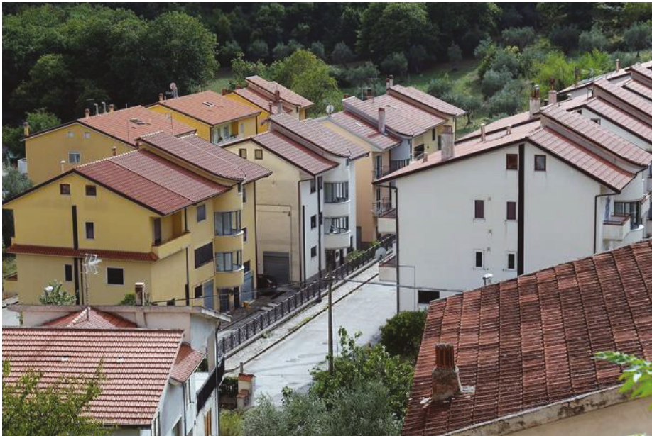
Figure 93. Salvitelle: details of new buildings (photos by [35,36]).
