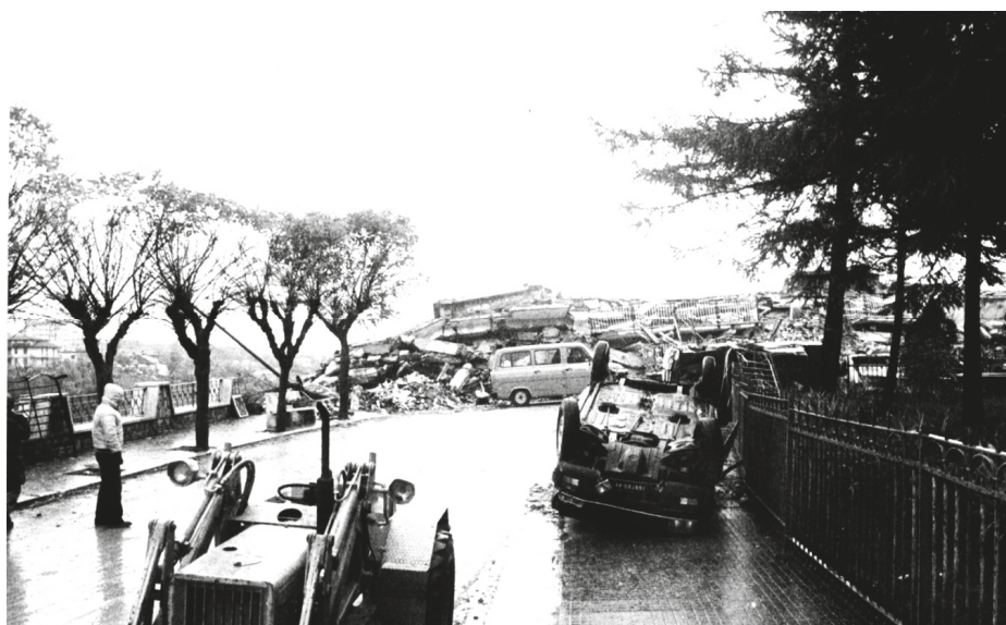
Figure 3. The earthquake in Sant'Angelo dei Lombardi. On the background, the “pancake effect” (Courtesy of Michele V.).
