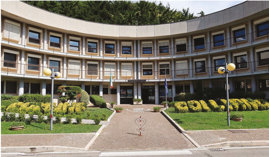
Figure 80. Colliano: the new Town Hall of the village (photos by [35,36]).
