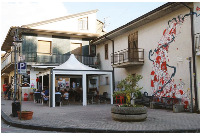
Figure 65. San Michele di Serino: detail of Cotone Street in which there were phenomena liquefaction triggered by the earthquake [22], (photos by [35,36]).
