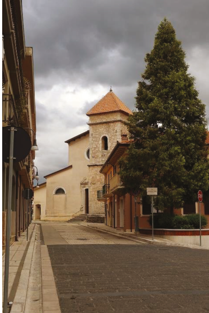
Figure 28. Lioni: restored Church and bell tower of S. Maria Assunta (photos by [35,36]).
