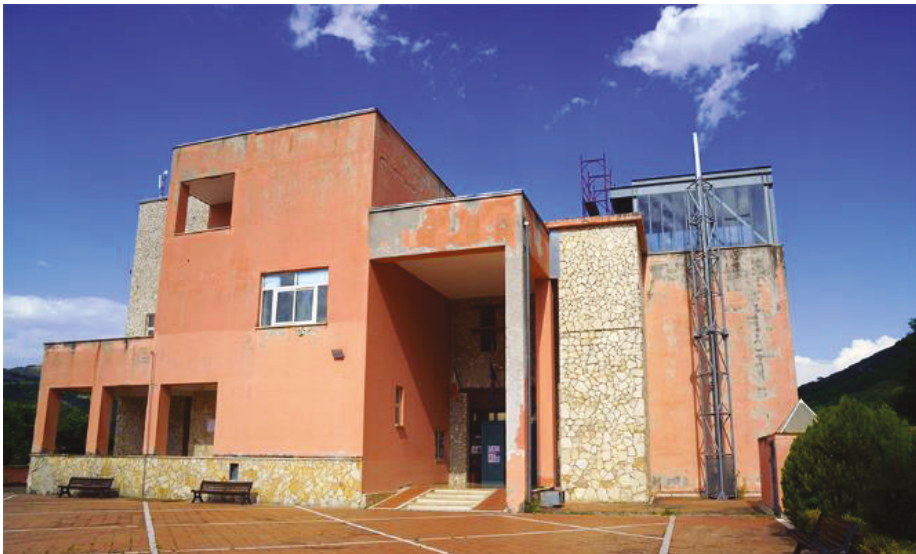
Figure 21. Laviano: the new Town Hall of Laviano (photos by [35,36]).
