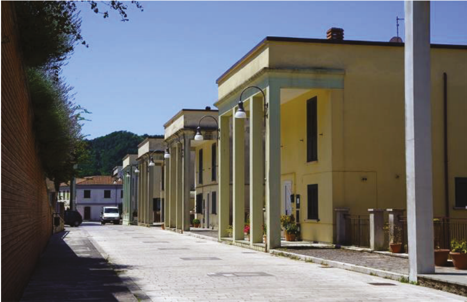
Figure 104. Teora: new reinforced concrete houses (photos by [35,36]).
