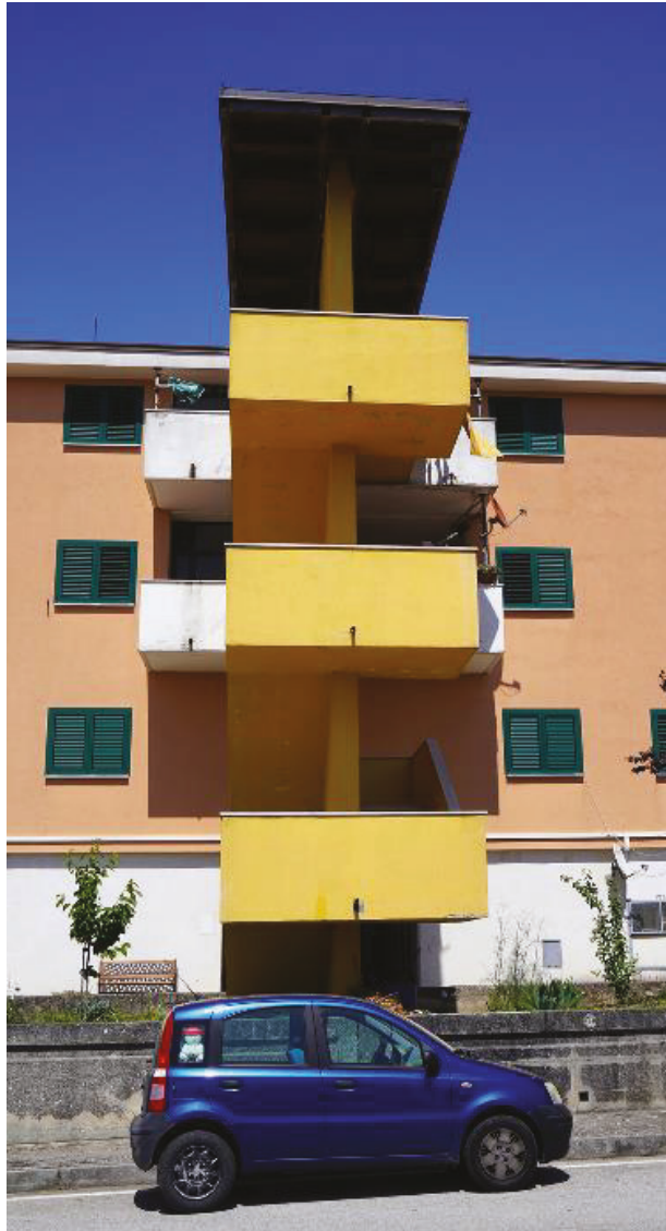
Figure 9. Castelnuovo di Conza: detail of new reinforced concrete buildings (photos by [35,36]).
