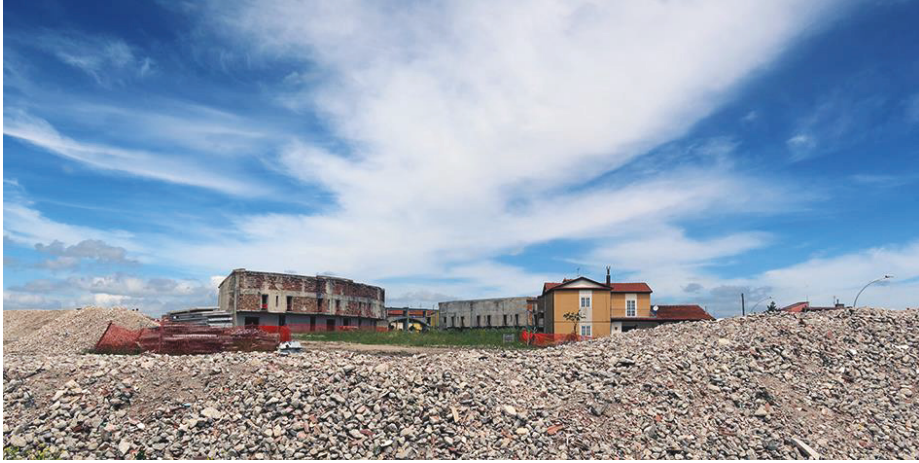
Figure 108. Bisaccia: the new village (Piano di Zona) with the remains of the new social housing still to be completed (Istituto Autonomo Case Popolari-IACP). A part of them has been demolished in 2020 (photos by [41]).
