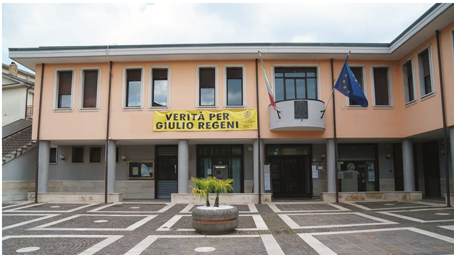
Figure 61. San Michele di Serino: the new municipal building (photos by [35,36]).
