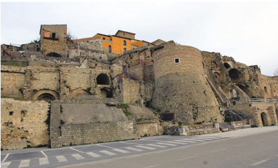
Figure 112. Calitri: historical centre, remains of some buildings that were recovered after the 1980 earthquake (photos by [35,36]).
