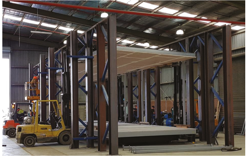
Figure 8. Forklifts handling partly finished modules within an offsite manufacturing facility.
