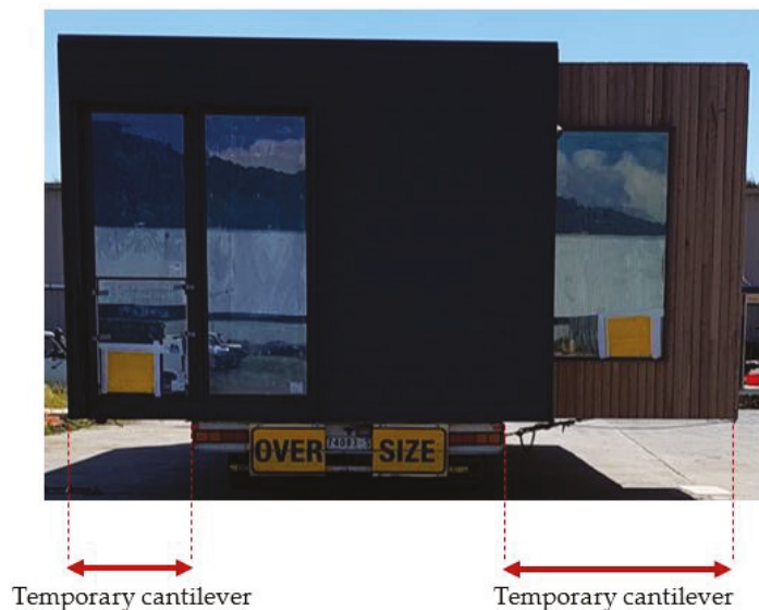
Figure 5. Temporary support conditions—An example of a situation where cantilevers which would not be there in the final state of a structure are imposed on a module during transportation.
