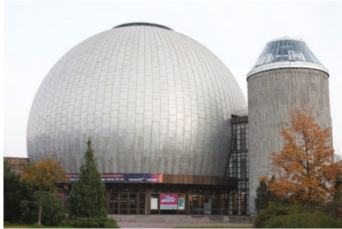
Figure 1. The Zeiss planetarium observatory, Berlin, Germany [1]. A hexagonal grid was used in order to create the spherical structure, called geodesic dome.
