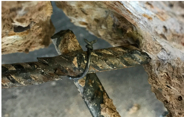
Figure 14. Plastic deformation of flexural tensile steel reinforcement in the cantilever section of S6 (photo by IMB, RWTH Aachen University).
