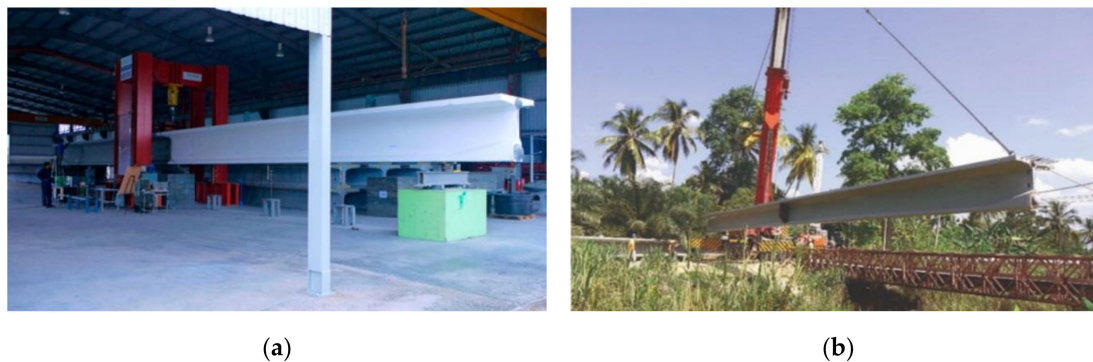
Figure 7. (a) Full-scale destructive test on a 30 m long segmental T-beam, research done in 2007–2010 [14,15]; (b) construction of 30-m-span Ulu Chemor bridge, stitched T-girder construction [15].
