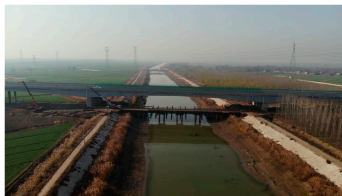
Figure 1. Photo of Xiaoqing River Bridge.
