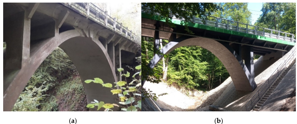
Figure 1. Jagodnik arch bridge before (a) and after (b) reconstruction.
