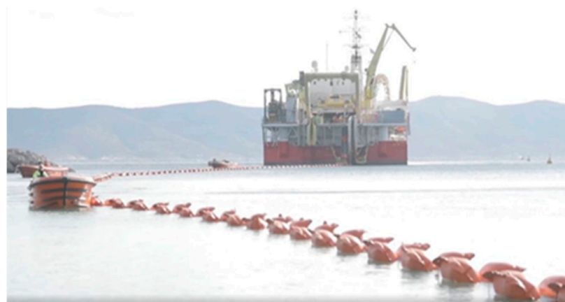
Figure 3. Floaters for submarine cable landing. Adapted from [34].
