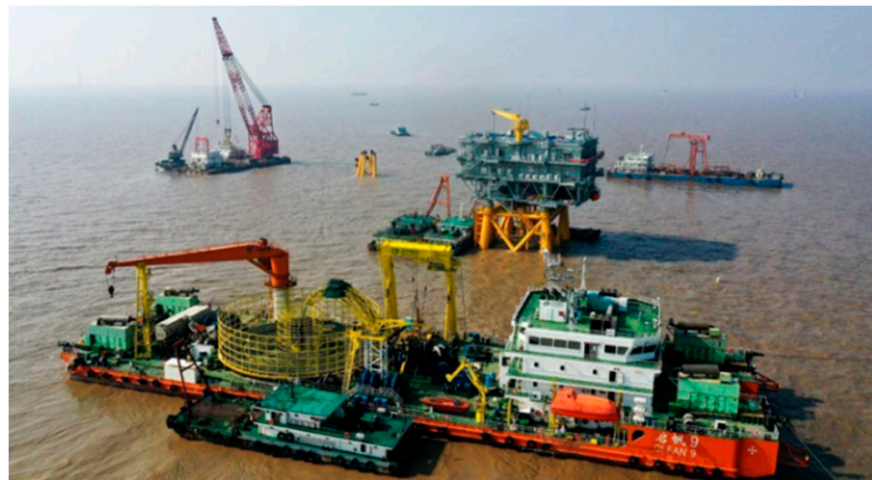
Figure 1. Qifan No. 9 cable-laying vessel.
