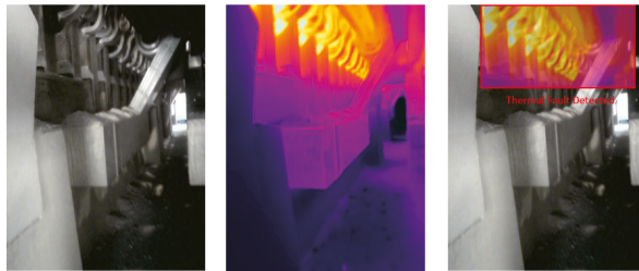
Figure 26. Thermal anomalies detection on-site for test run 4.
