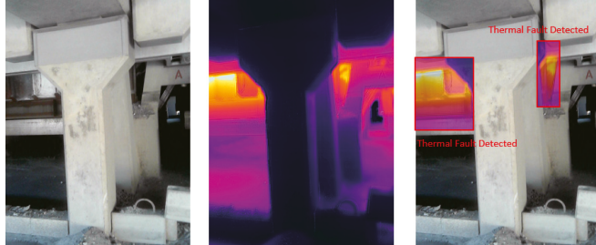
Figure 24. Thermal anomalies detection on-site for test run 2.
