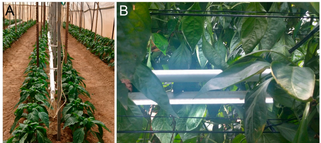
Figure 1. Intra-canopy supplemental illumination. (A) Installation of the 'Bioled' light fixtures at the center of the beds (September 2019, prior to start of illumination treatments). (B) Side-view of intra-canopy back-to-back LED illumination (picture acquired in March 2020).
