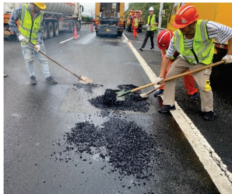
Figure 6. Manual milling hot pavement.
