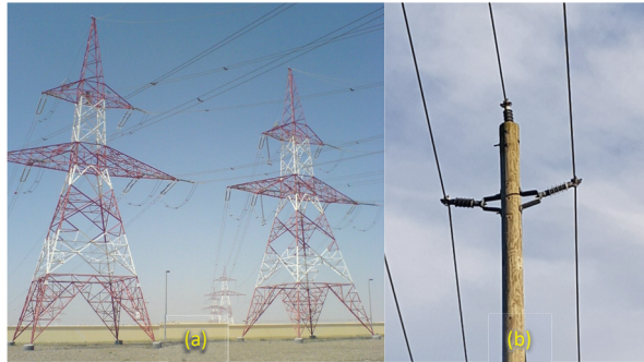
Figure 10. Photos of (a) a 220-kV overhead transmission line where outdoor insulators are employed to electrically isolate the conductors from the grounded towers, and (b) is a 12.47-kV wooden post using polymer insulators for isolating the conductors from the pole.
