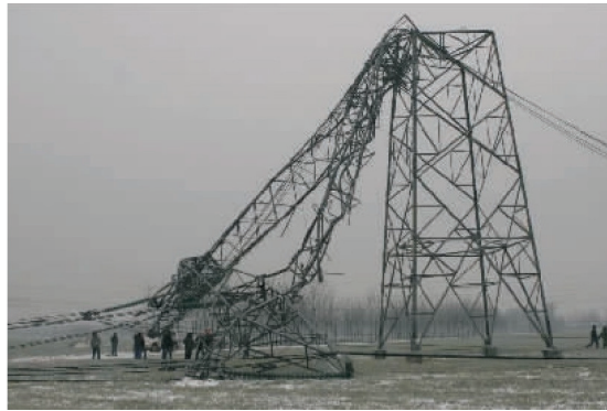
Figure 1. The collapse of the power grid tower was caused by the snow and icing disaster [10].
