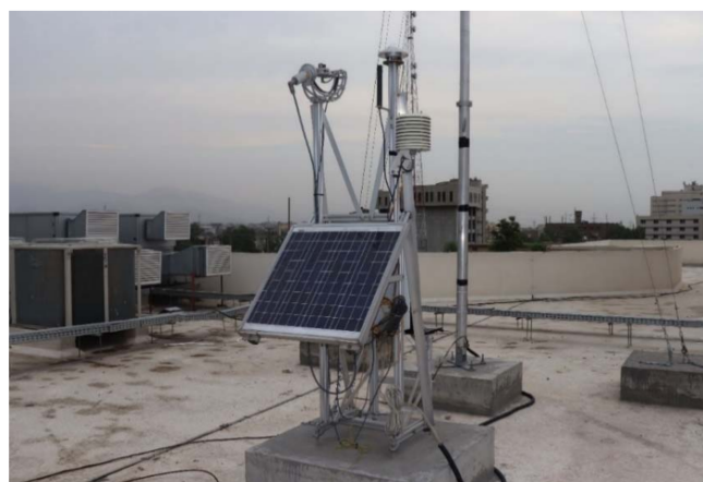
Figure 1. Weather Station established at UET Peshawar.
