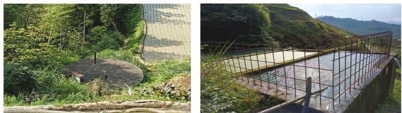
Figure 3. One of the Cistern and Sewage Treatment Centres in Ping'an (Source: by author 1).
