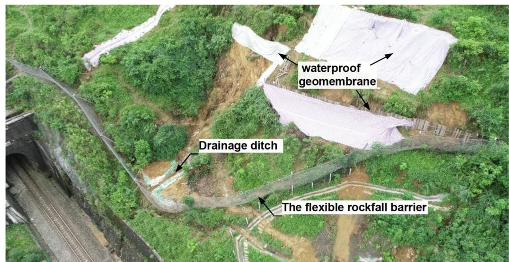
Figure 5. An overall view of the landslide site after maintenance.
