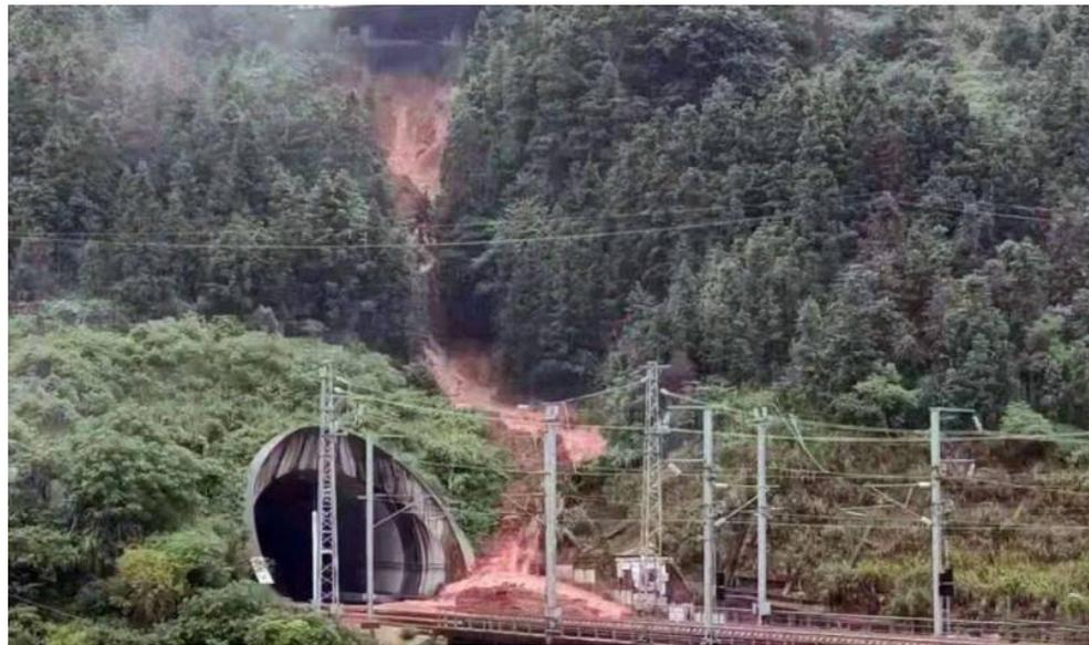
**Figure 1.** Landslide debris occurring near a high-speed railway tunnel exit [9] (Rongjiang, Guizhou, China).
