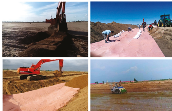
Figure 2. A typical sequence of agricultural land preparation: excavation, Breathable Sand layer preparation, backfilling, and planting.
