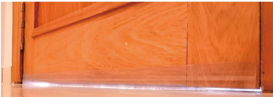
Figure 9. Weatherstripping to improve the thermal insulation of the house.
