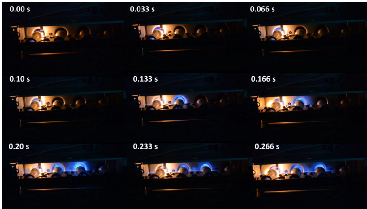
Figure 15. Rolling ignition of a non-condensing furnace at a 30% H 2 blend.
