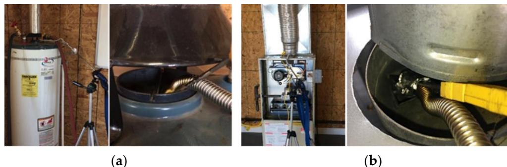
Figure 7. Field-testing exhaust sampling examples for: (a) water heaters; (b) furnaces.
