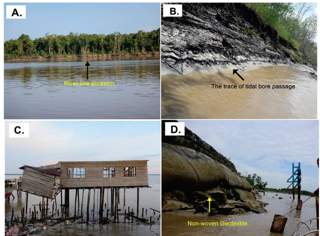
Figure 9. The impact of tidal bore propagation on the surrounding environmental conditions. River-line abrasion (A); coastal erosion at the edge of the river (B); local settlement destruction due to tidal bore (C); non-woven geotextile fabrics as coastal protection applied in several areas of interest (D).
