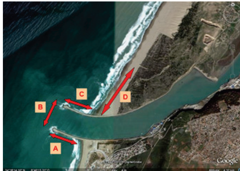
Figure 5. The different zones subject to analysis: stress on structures (A, C), B-agitation in the river outlet (B), littoral erosion (D).
