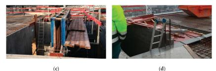
Figure 4. Observations collected during the inspection at the project: (a) a barrier is missing on one of the floors of the building; (b) an unsafe opening on the staircase shaft; (c) missing barriers on the central core of the building; and (d) an opening not covered with barriers. (Own source).
