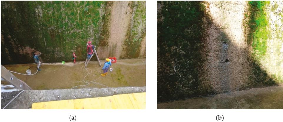
Figure 3. Investigation of the civil engineering works of a dam (a) and the current state of its concrete (b).
