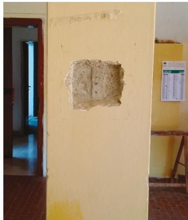
Figure 4. NDTs: preparation for Hammer Test and Ultrasonic velocity Test.
