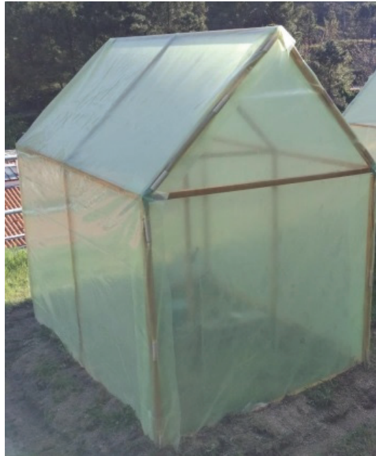
Figure 2. Picture of the greenhouse with the polyethylene cover applied.
