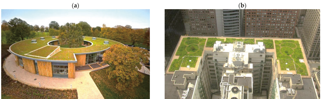
Figure 2. Examples of green roofs: (a) British Horse Society Headquarters, UK, and (b) Chicago City Hall, USA [31].
