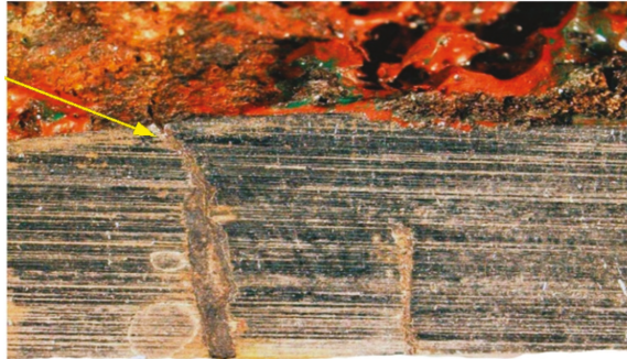
Figure 22. The passage of the crack from part II into part I through the weld that joins the two parts (handy-size bulk carrier 30206 DWT). Macroscopic examination.
