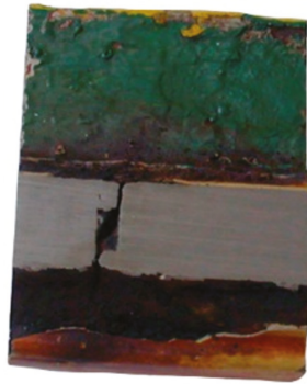
Figure 41. The merging of cracks previously branched at the bolt thread (handy-size bulk carrier 30185 DWT). Macroscopic examination.
