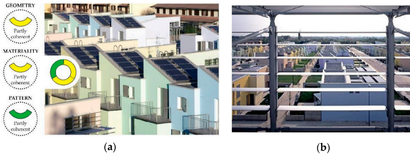
Figure 12. Architectural integration matrix for the PV systems at Violino District in Brescia (left); (a) system modular pattern (photo: © Fabio Cattabiani); (b) view from the roof of one of the multi-family houses (photo: © Fabio Cattabiani).
