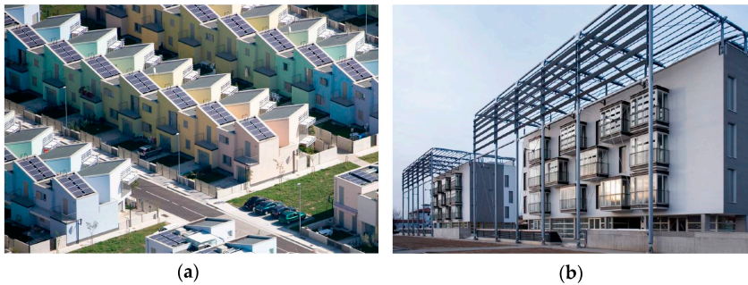
Figure 11. (a) Aerial view of the terraced houses of Violino District (source: © BAMSphoto—Basilio) and (b) the two multi-family houses (photo: © Fabio Cattabiani).
