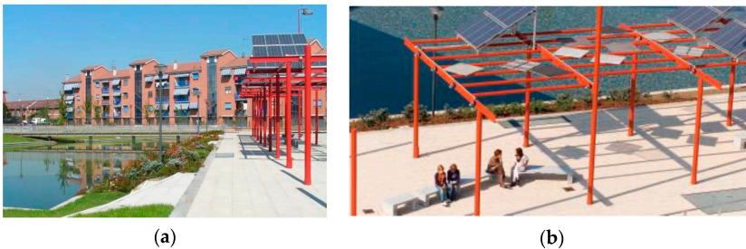
Figure 5. Ground (a) and aerial (b) view of the pergola equipped with PV panels in the public area (source: © Municipality of Alessandria).
