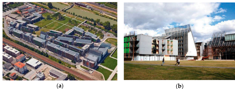
Figure 9. (a) Aerial view of the Le Albere district (source: © Google Earth) and (b) view from the public park (photo: © Silvia Croce).
