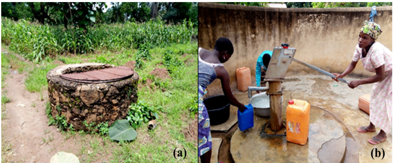
Figure 4. Traditional sinks exploiting the water of the alterite reservoir at Niamtougou (northwest of the study zone) (a) and borehole equipped with a human-operated pump, exploiting the water of the fractured reservoir at Bébéda (center of the study zone) (b).
