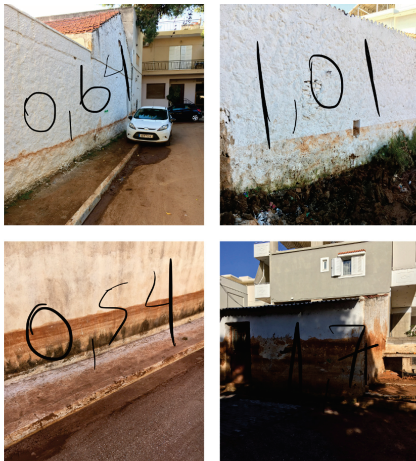
Figure 4. Indicative observation points in Mandra town (in roads): the observed maximum depths are 0.64 m (up & left), 1.01 m (up & right), 0.54 m (down & left), 1.70 (down & right).
