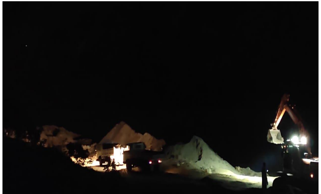
Figure 4. Sand Extraction near the Neelam Riverbed, Muzaffarabad.
