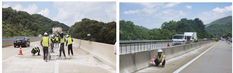
Figure 14. Workers working on the road during observations for research.
