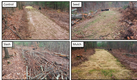
Figure 3. A comparison of the four skid trail closeout best management practices (BMPs) used in the study.
