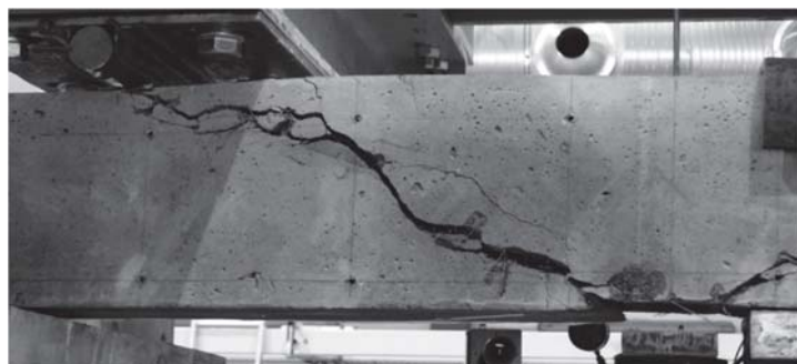
Figure 17. Example of a shear tension failure in the shear area of BF series beams.
