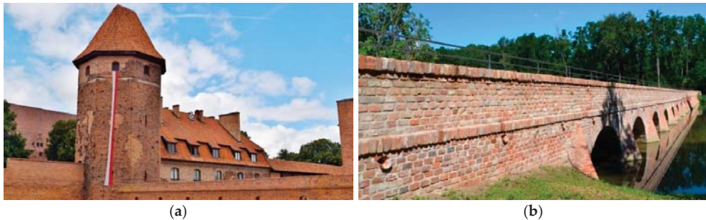
Figure 1. (a) Reconstruction of the Gothic castle in Malbork (Poland) with modern masonry elements, (b) Reconstruction of a baroque brick bridge near Mikulov (Czech Republic) with historical masonry elements.
