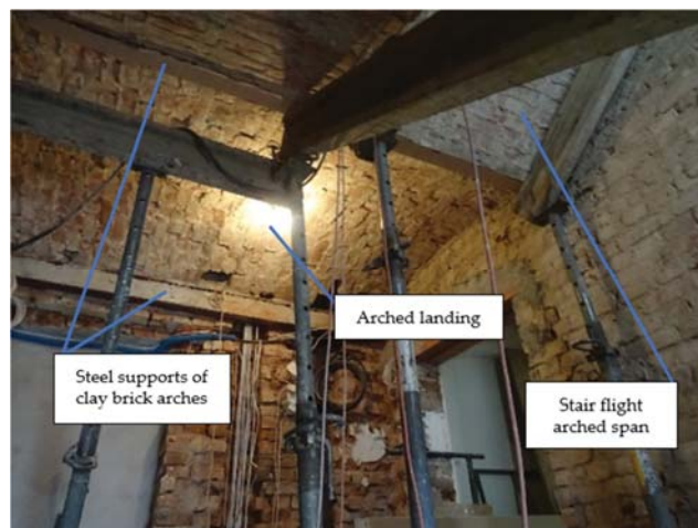
Figure 5. View of the researched masonry staircase.
