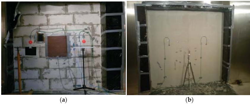
Figure 3. Photo of tested building enclosure (in this case, insulated wall A) with visible arrangement of sensors: (a) on warm chamber side, (b) on cold chamber side.
