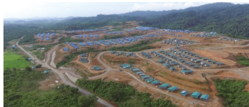
Figure 4. Resettlement site of Payit Village with green roof and Yegauk with blue roof.
