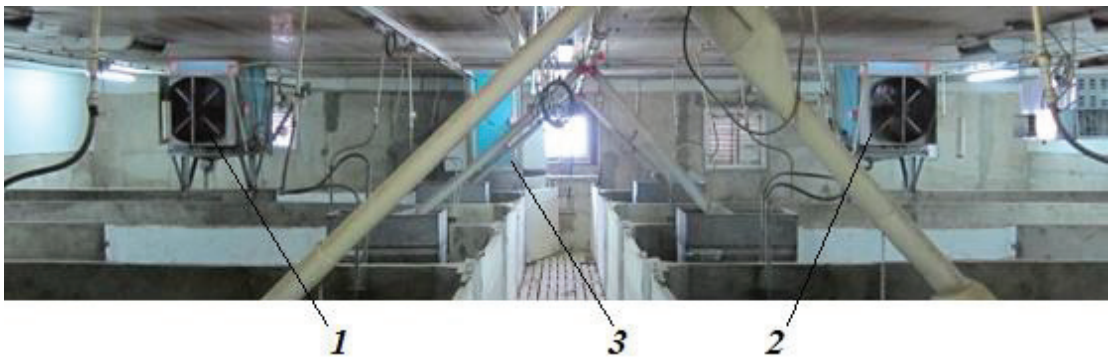
Figure 10. General view of the experimental system of climate control inside the pig house: 1,2—UT-6000C unit (for general exchange ventilation); 3—UT-3000 unit (for air extraction from the manure channel).
