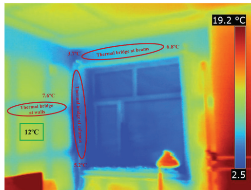
Figure 16. Thermal imaging of the benchmark building's northwest position.
