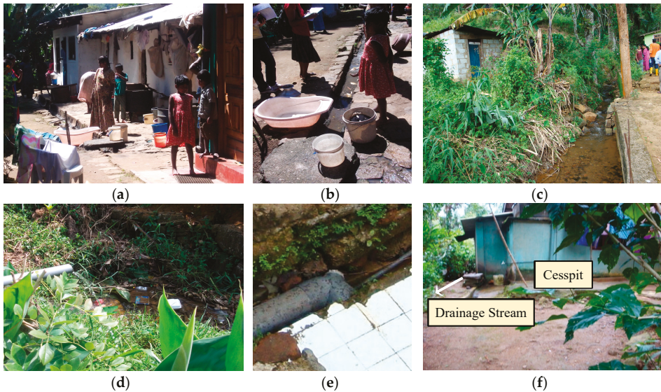
Figure 2. Photographs of the environmental conditions at locations in the study area. (a) A congested row of line houses. (b) A polluted drain which flows to the stream. (c) A pit latrine close to the drain. (d) Wastewater disposal to the drain through a pipe line. (e) Septic tank effluent directed to the stream. (f) A cesspit close to a drainage stream.
