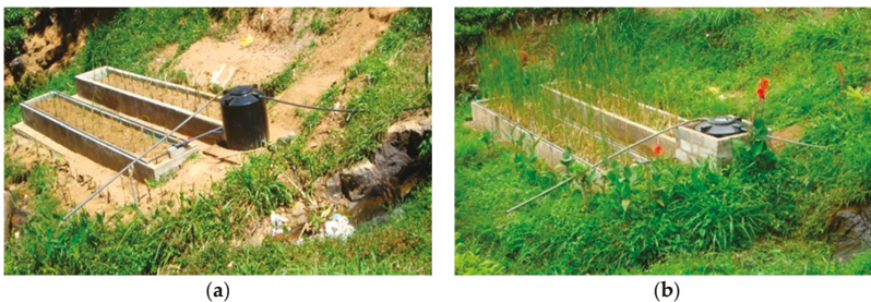
Figure 4. Arrangement of wetland units in the field: (a) just after planting; and (b) mature wetland units.
