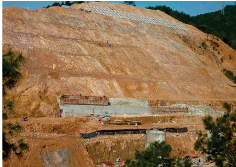
Figure 2. The high cutting slope of section DK592 + 532.00~ + 562.00.
