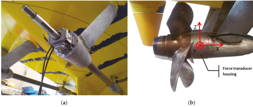
Figure 3. (a) installation at the tail shaft (b) final configuration.
