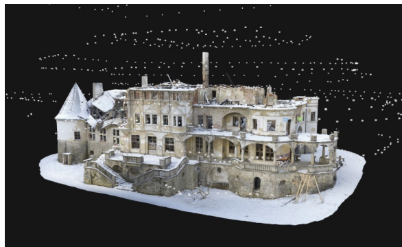
Figure 8. Aerial photogrammetry positions.
