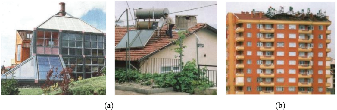
Figure 1. (a) The Chanelle house, Stavanger, Norway was one of the first modern energy autonomous buildings in Europe trying to integrate renewables like solar PV, solar thermal, windmill and battery and thermal storage in a more architecturally acceptable way through building integration. The house designed by the author was an attempt at showing alternatives to the messy roofscape developing throughout Europe at the time, due to lack of engagement among architects, as this picture from the Eastern Europe apartment block and the Greek house show the roof chaos is total (b). All photos: the author.
