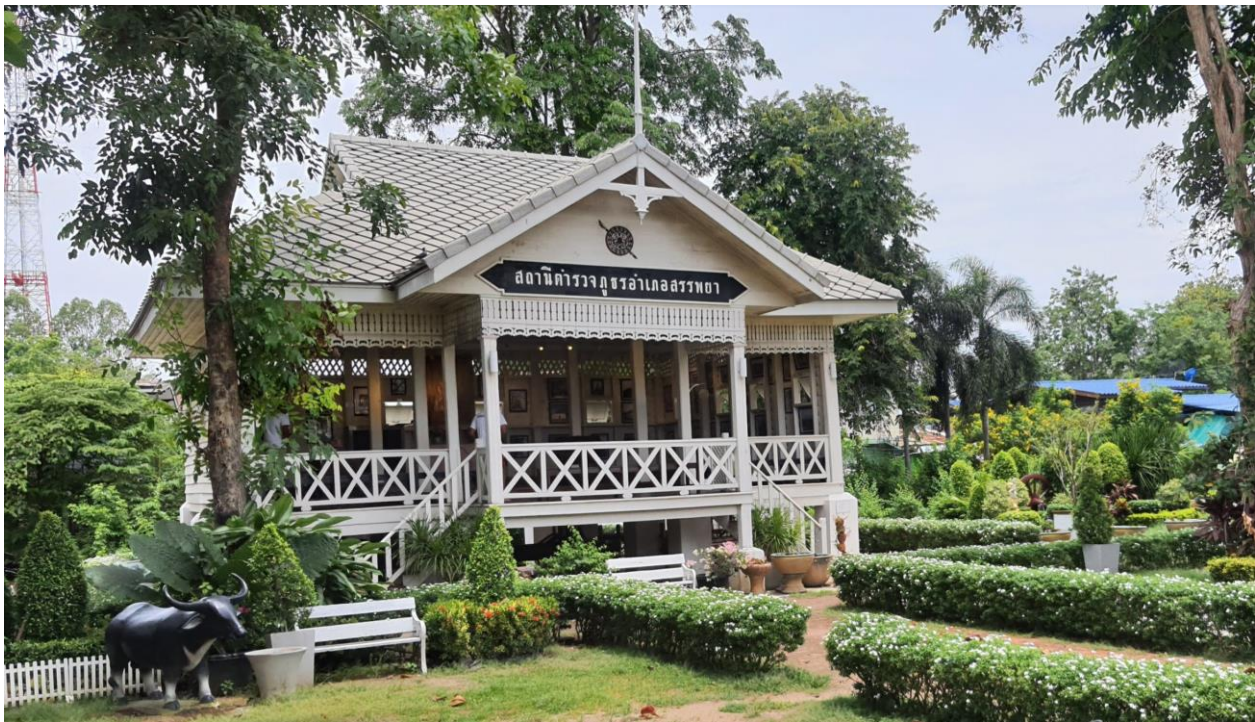
Figure 3. The old police station of Sapphaya. Source: authors' photo.
