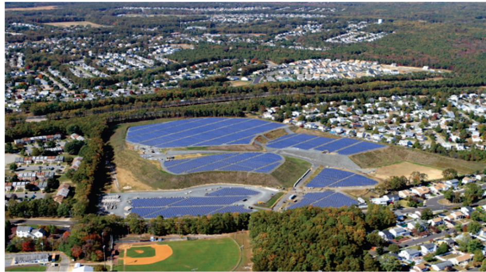
Figure 8. Brick Town landfill. Solar panel view [38].
