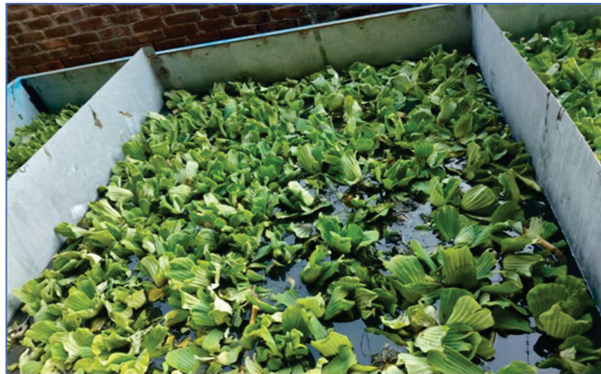
Figure 3. Water lettuce in the Sialkot floating treatment wetland (photo: A. Youns and J. Shafiq).
