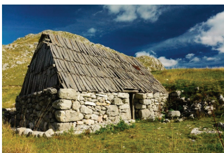
Figure 22. Glada with larger and better-dressed blocks—Upper Rikavac, the katun of Dučići, photo: I. Laković.
