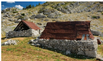
Figure 31. Glada’s roof made of the tin barrels—Koštica, Kotski katun, photo: I. Laković.
