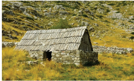
Figure 17. Gladas with its faces oriented perpendicularly to the terrain, partially dug into the ground—Koštica, Kutski katun, photo: I. Laković.
