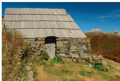
Figure 20. Construction of slate, photo: I. Laković
