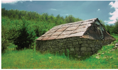
Figure 16. Glada with its face oriented parallel to the terrain, partially dug into the ground—Građen, Podgradski katun, photo: I. Laković.
