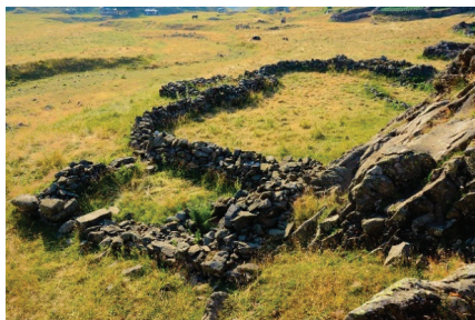
Figure 33. Sheep corral ( torina ) built in drystone—Bušat, photo: I. Laković.
