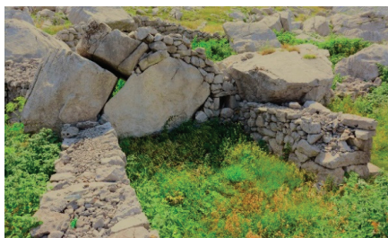
Figure 14. Existing rocks and larger blocks of stones were used for parts of gladas' walls. Studenica, photo: I. Laković.
