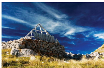
Figure 24. Roof construction of the glada with rafters, Momonjevo, photo: I. Laković.
