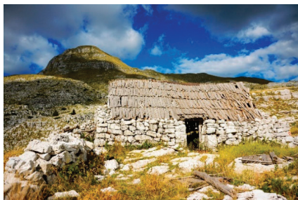
Figure 29. Roof cover of skudla —Bankanjski katun, photo: I. Laković.
