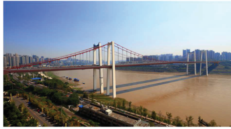
Figure 1. Egongyan rail bridge.
